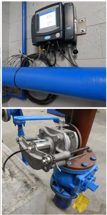
RAS/WAS room showing Solitax TSS probe in place.
