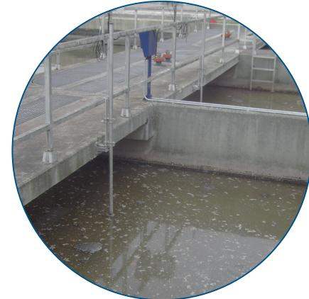
Fig. 5: Simple installation thanks to variable fitting systems. The best measuring point depends on the hopper design and must be determined by carrying out comparative measurements.
