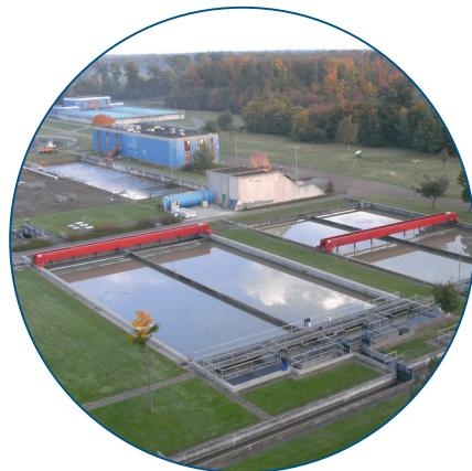
Fig. 1: Link between biological treatment and sludge treatment – primary settlement tanks.
