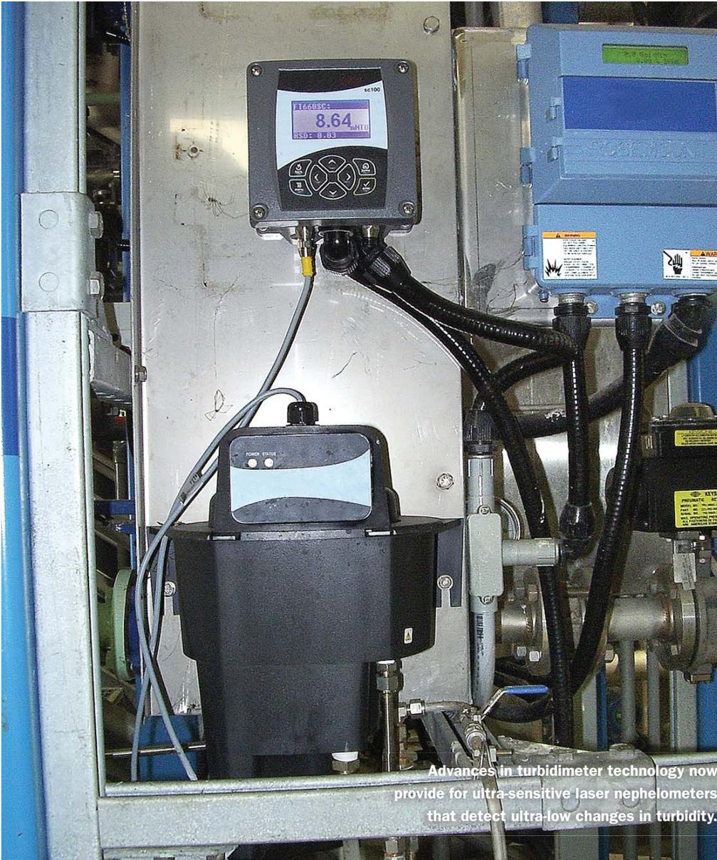
Advances in turbidimeter technology now provide for ultra-sensitive laser nephelometers that detect ultra-low changes in turbidity.
